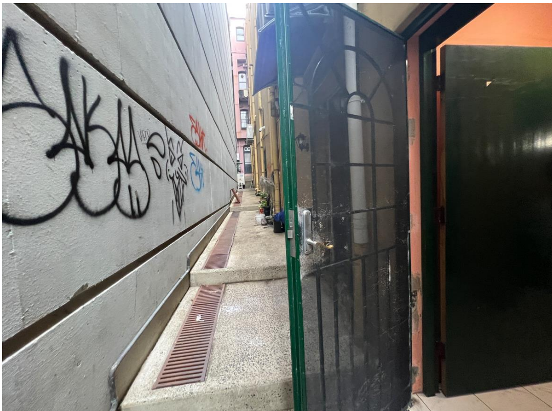
Figure 8: Rear accessway from Kent Street facing east to the subject site
