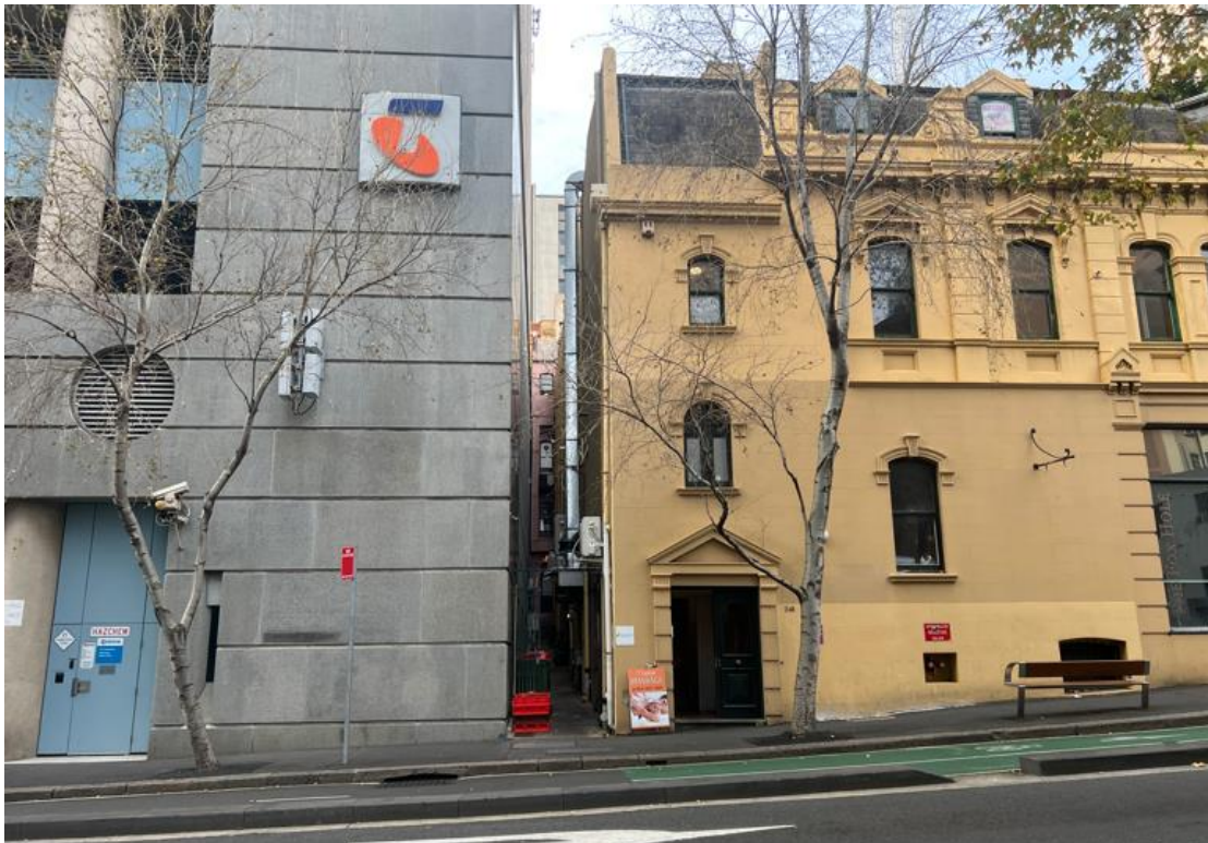
Figure 4: Rear access to the subject site from Kent Street between 97-105 Clarence Street (left) and 68A Erskine Street (right) facing east
